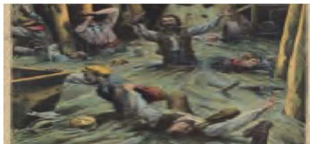
Figure 10: Collapse of the Kandersteg Tunnel
